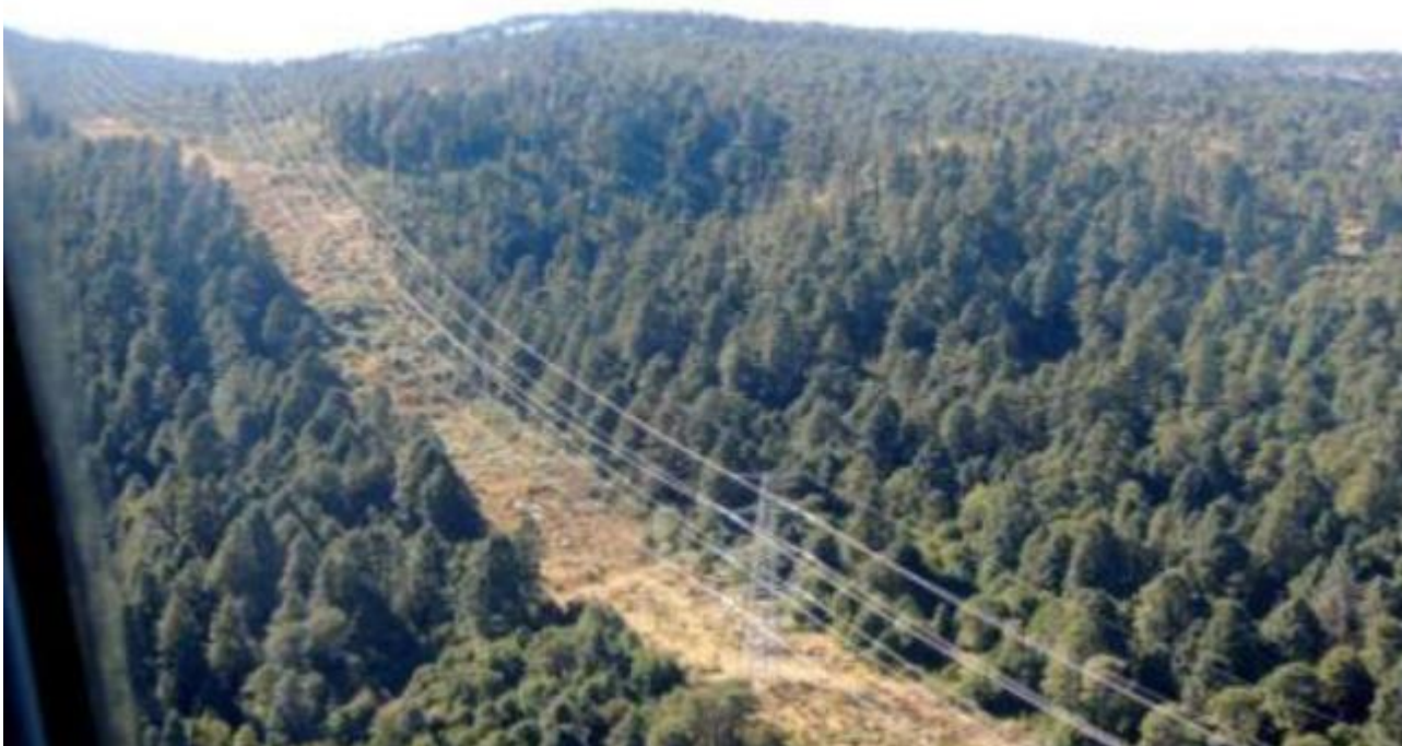
Figure 3.3 – Panoramic view of right-of-way in a 400kV overhead line
