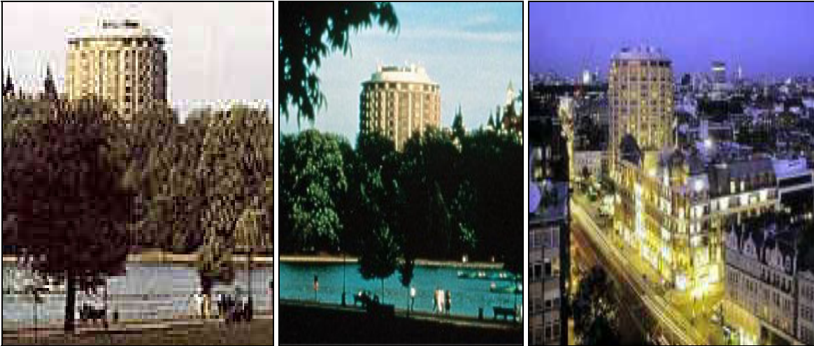
Figura 13.6. Sheraton Park Tower
